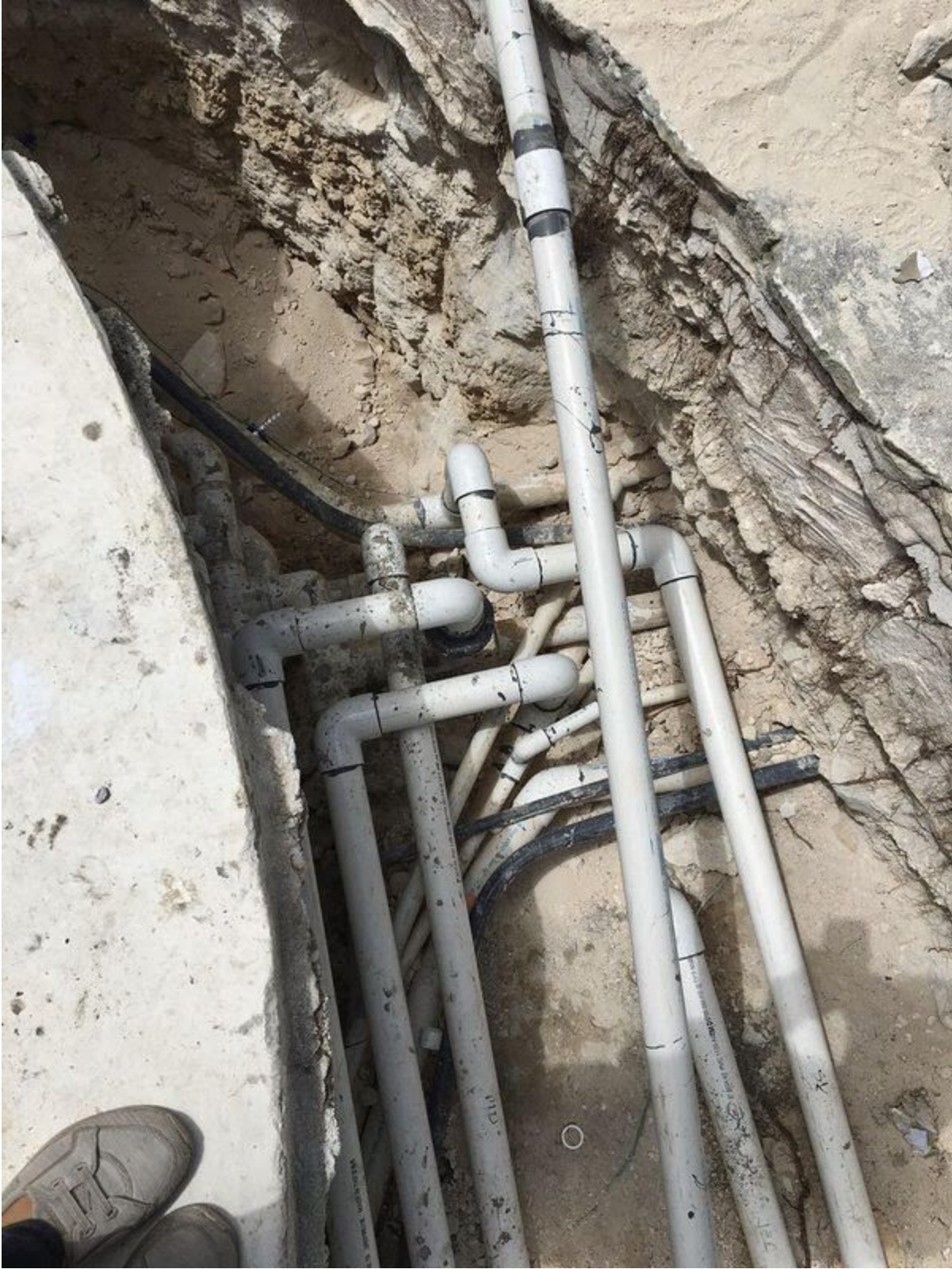
Hot tub trenching and dig out.
