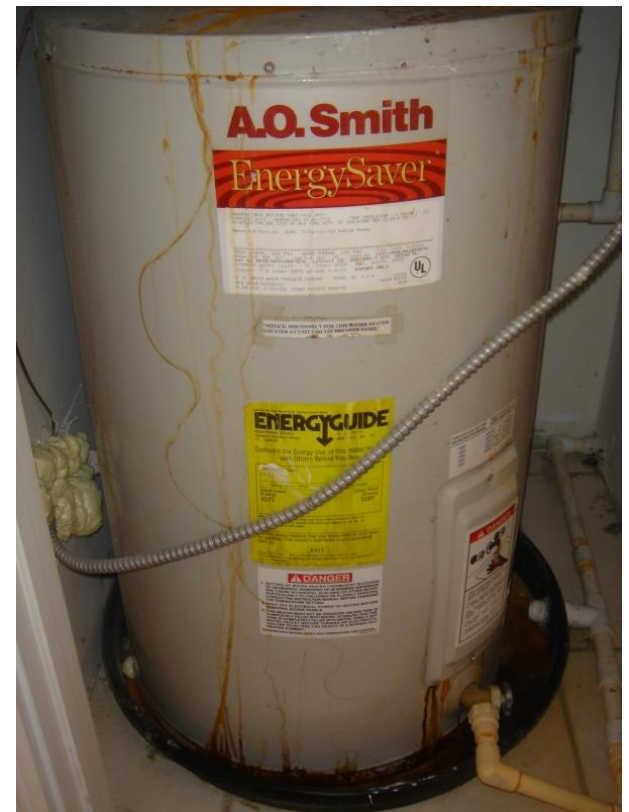
Water Heater replacements
