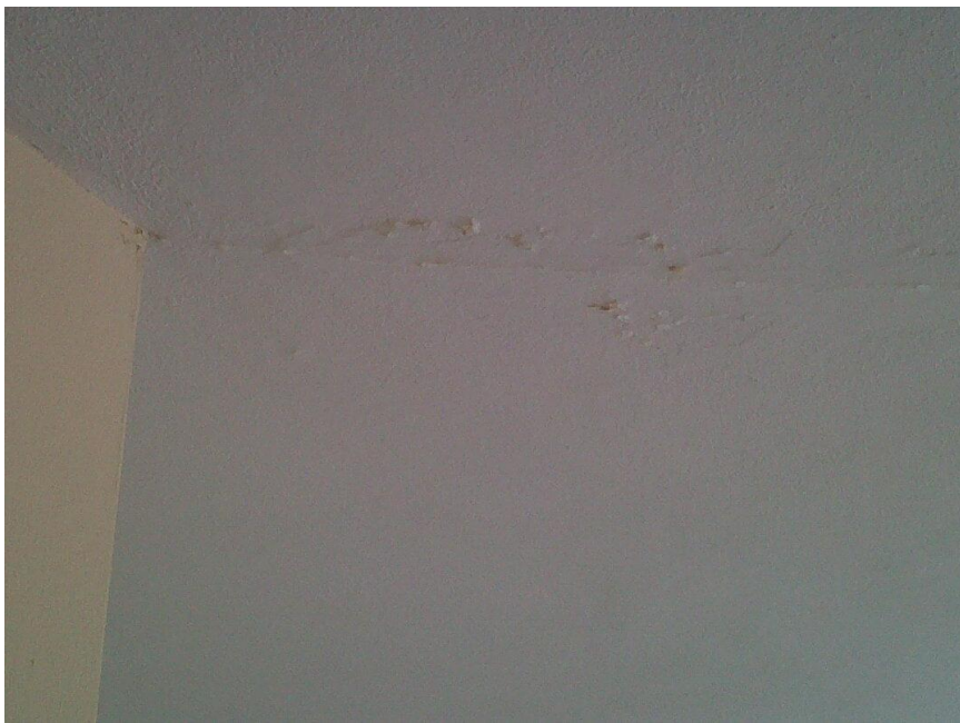
Damaged ceilings in Owners' Units – mold, bubbling & water
