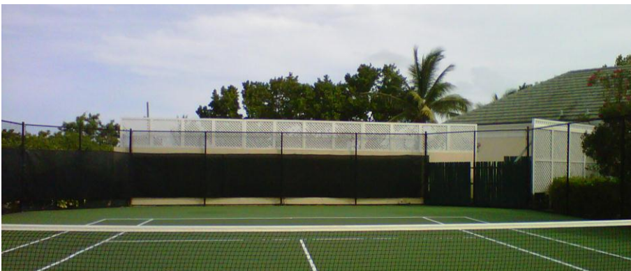
Tennis Court – Lattice Coverage
