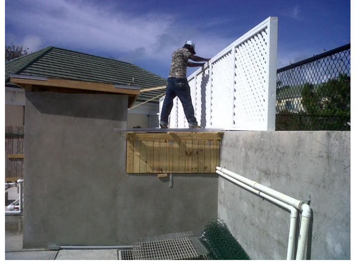
Tennis Court – Lattice Coverage
