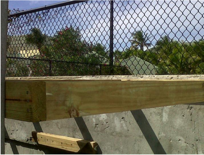
Tennis Court Fencing
