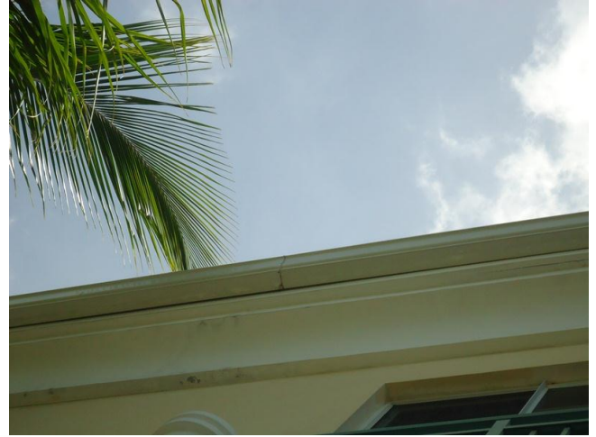
Gutters Repairs – Building 5
