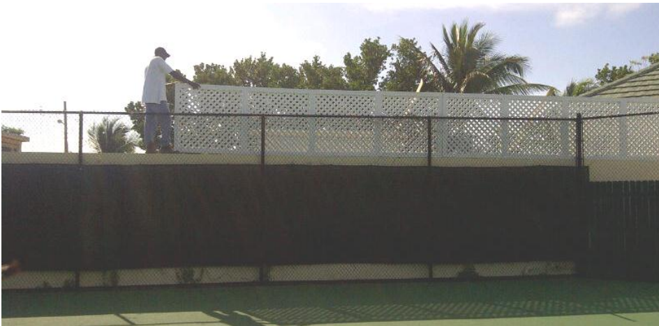
Tennis Court – Lattice Coverage
