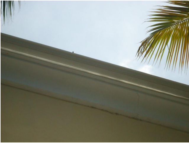
Gutters Repairs – Building 4
